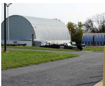
Airfield Maintenance Building Image by Delta Airport Consultants
